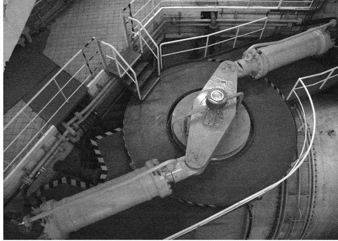
Figure 2.2: Closed loop with  $I_0$  controller equivalent to the structures from Fig. 2.1 (above) and example of hydraulic actuators with I character (below).
